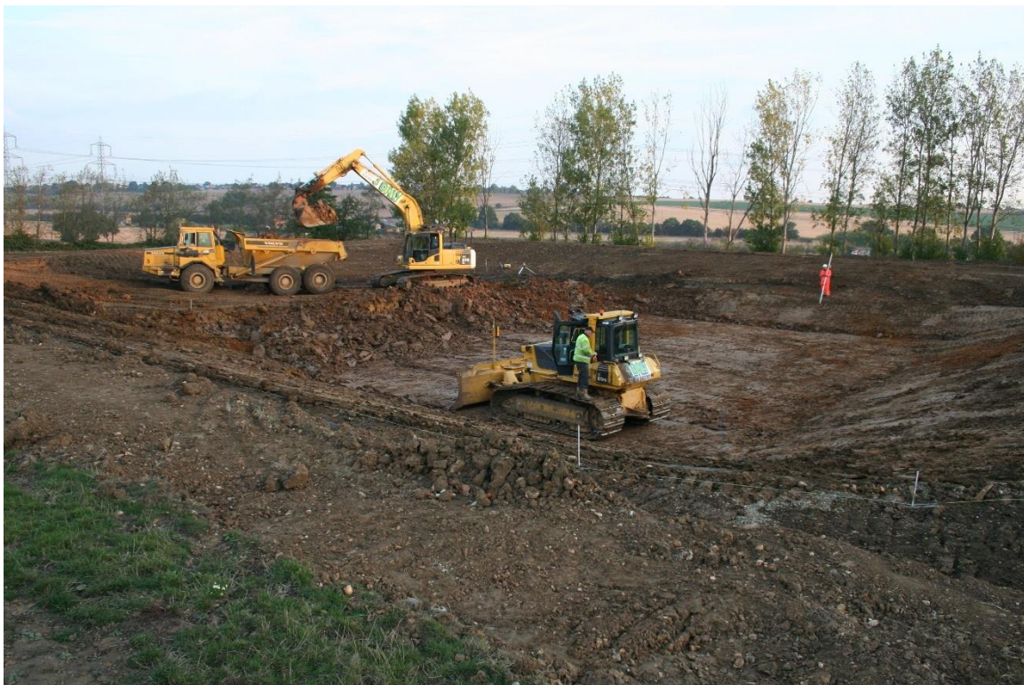
Excavating the flood storage lagoon (image shows the depth of the lagoon for the flood storage area)
