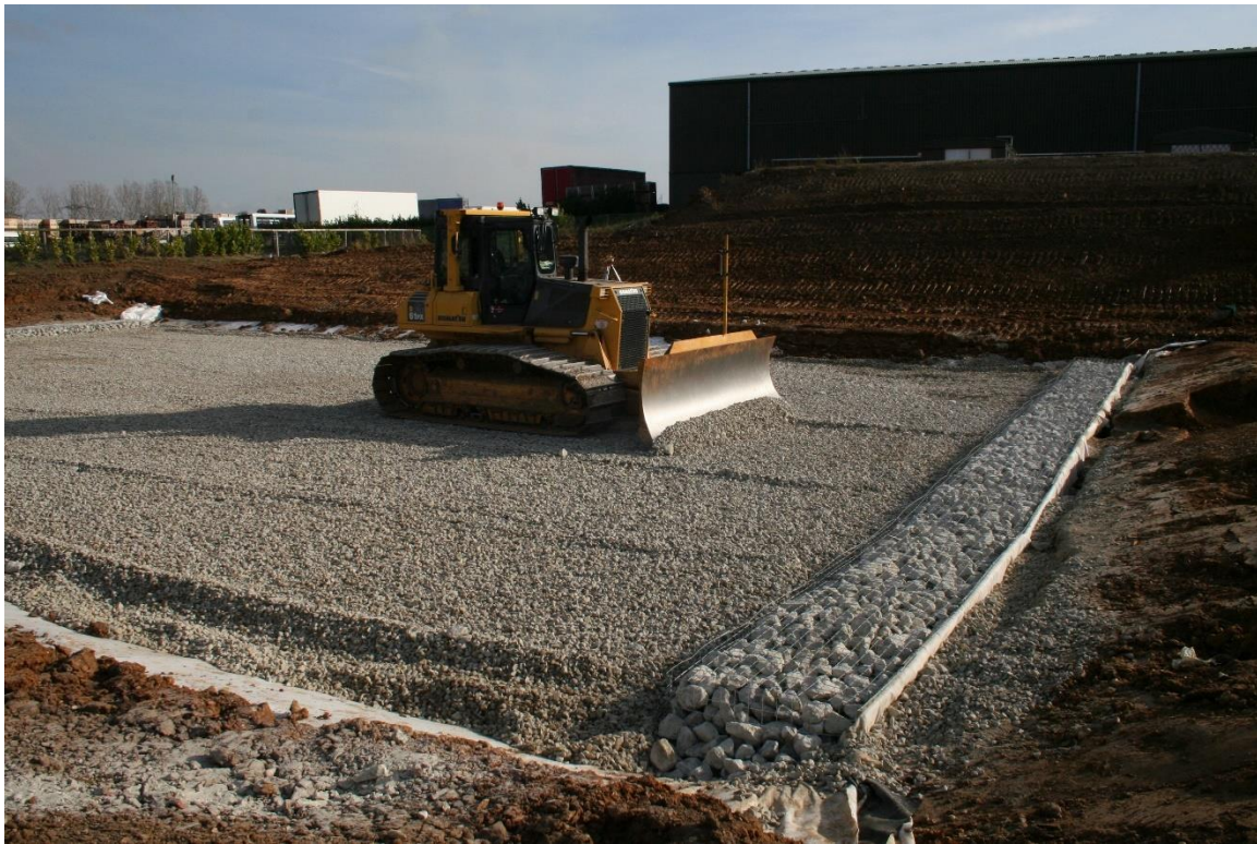
Excavating three treatment beds (image shows the levelling of the beds)
